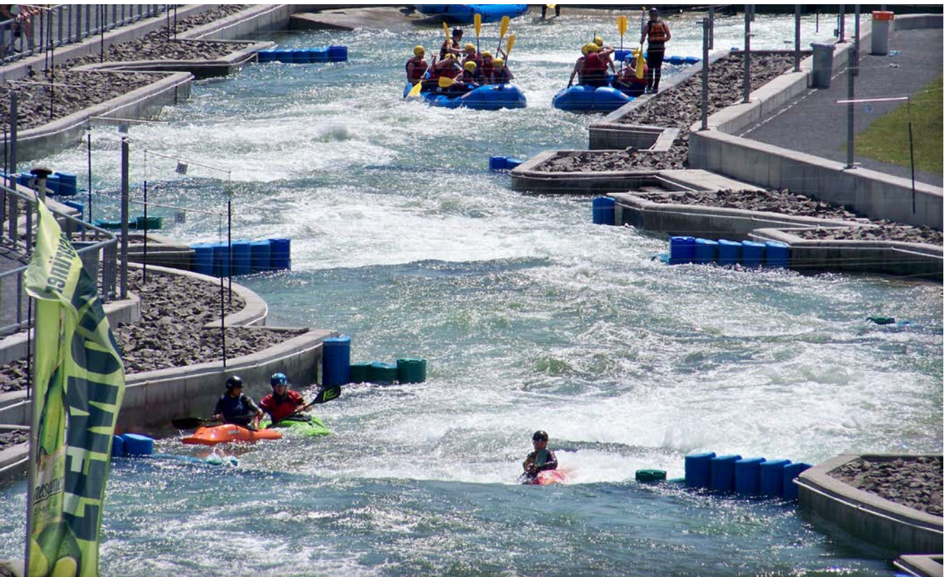
Assoziativbild: Markkleeberger See - Wildwasseranlage By Joeb07 (Johannes Kazah) - Own work, CC BY 3.0, https://commons.wikimedia.org/w/index.php?curid=16034364
