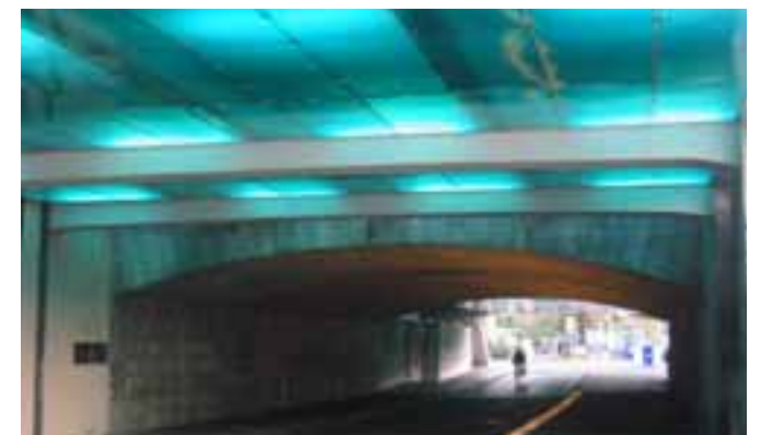
Lichtinstallation in Tunnel
